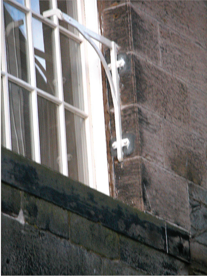
Figure 2. Gregory's telescope bracket placed in one of the southern windows of the rebuilt Upper Parliament Hall as seen from the Quadrangle of St Mary's College. The bracket head is 6.75 metres above ground level
